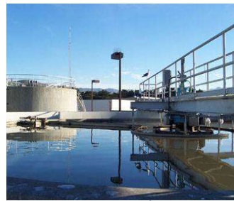
Construction / infrastructure / water management
