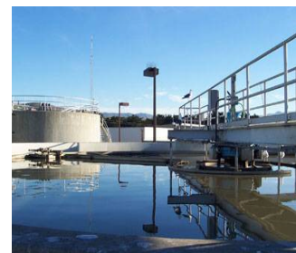
Construction / infrastructure / water management
