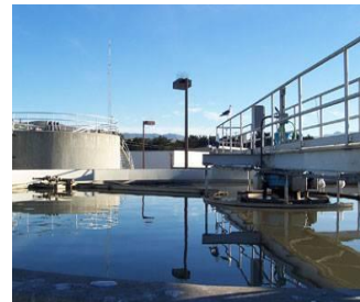
Construction / infrastructure / water management
