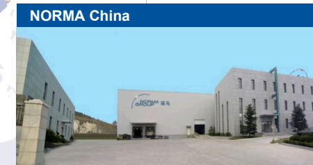
NORMA China Increase capacity to enable expansion
